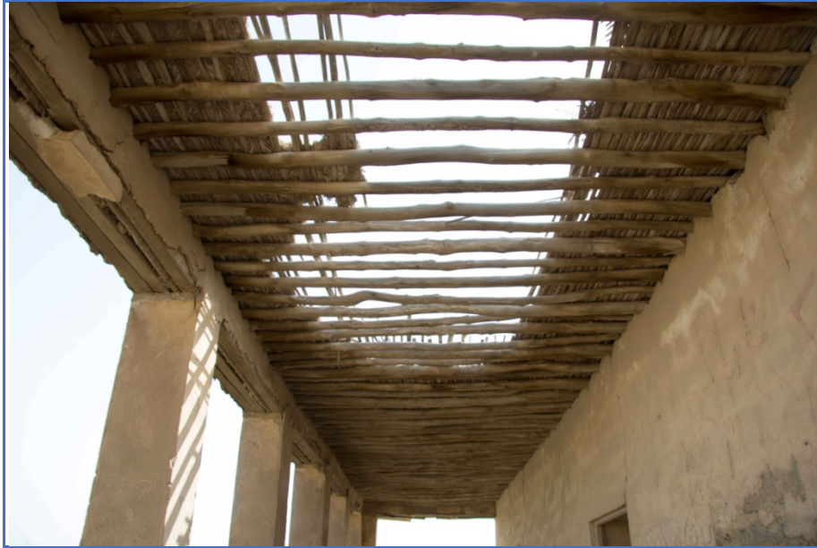
Figure 26: Round danshal roof timbers in the external liwan area.
