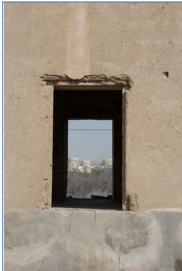
Figure 31: Window on the south side of the building
