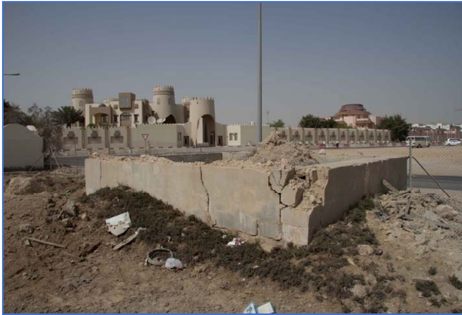
Figure 68: Concrete tank, Structure 7, looking northeast.
