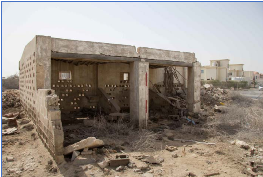
Figure 54: Stable block Structure 4, looking southwest.
