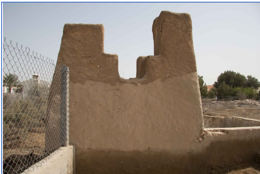
Figure 10: Photo of the west facing elevation of the well superstructure.
