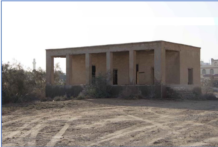
Figure 20: Majlis Structure 2 looking southeast.
