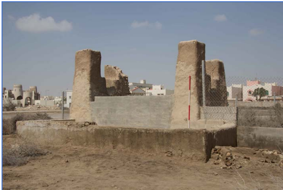
Figure 19: The well superstructure and water trough, looking north
