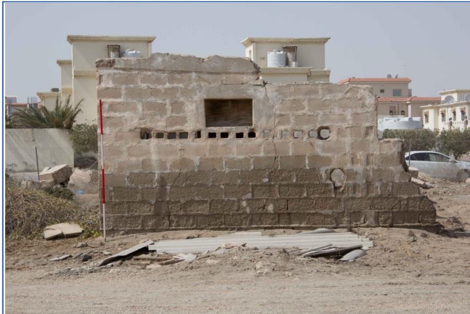
Figure 48: Photo of the west facing elevation of Structure 3.
