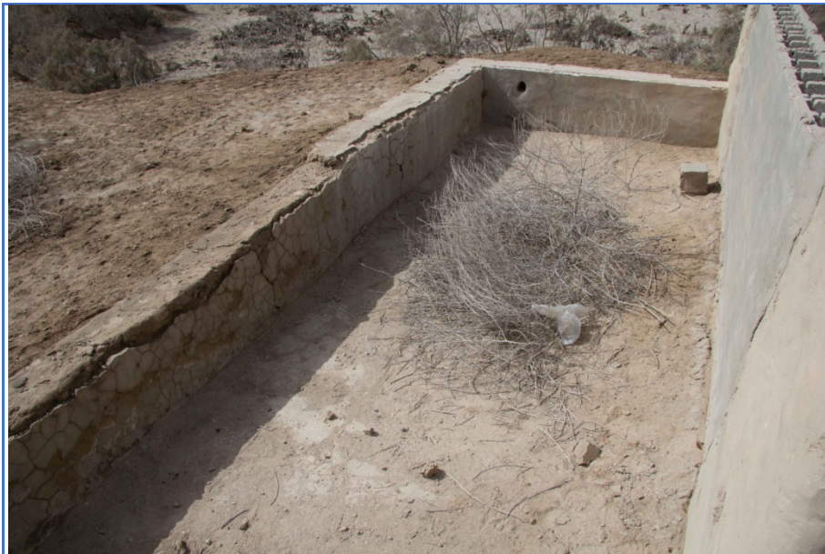
Figure 16: Water trough on the southern side of the well, the earlier phase of the trough is visible in the left foreground.
