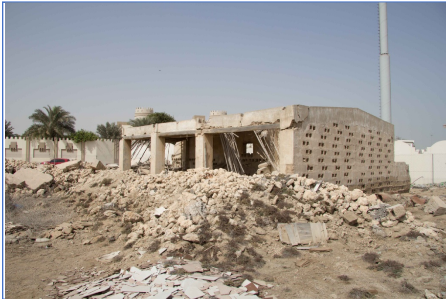
Figure 51: Stable block Structure 4, looking north west.
