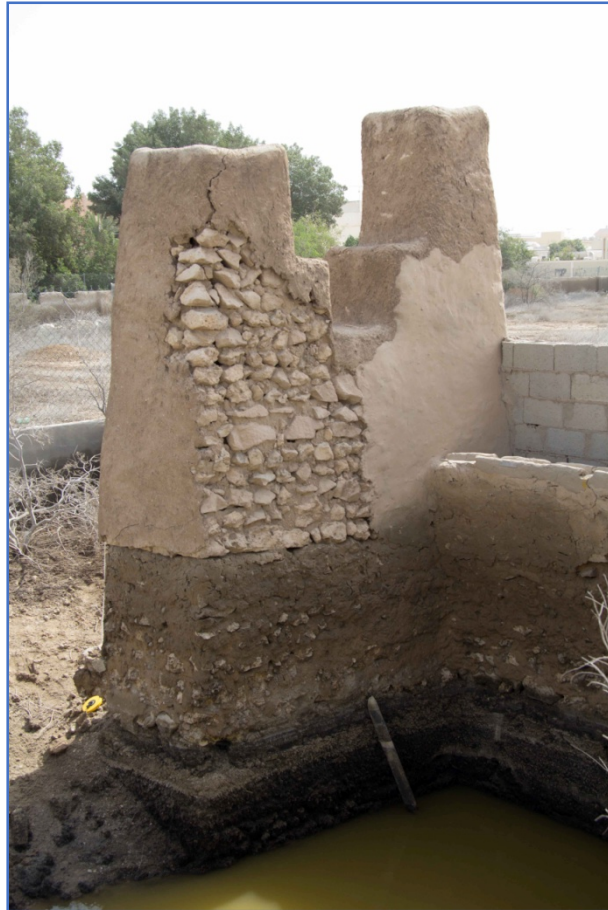
Figure 13: Construction of the well.
