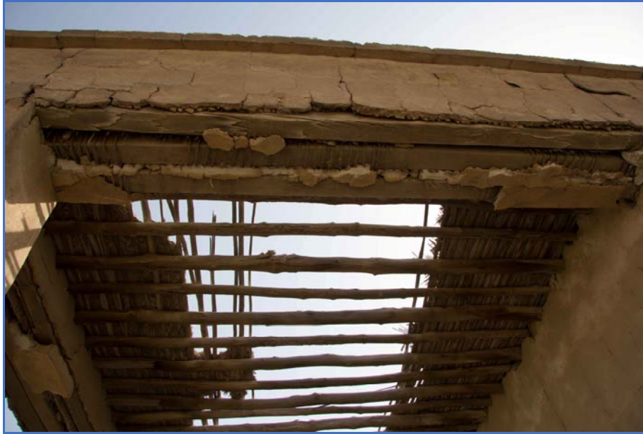
Figure 24: Detail of the construction of the colonnade.
