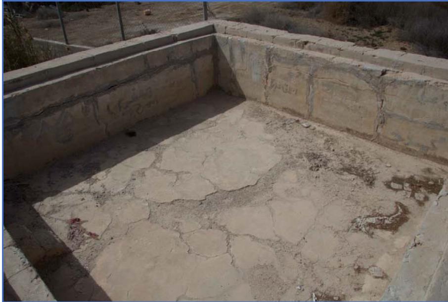
Figure 78: Internal view of raised tank associated with Structure 10
