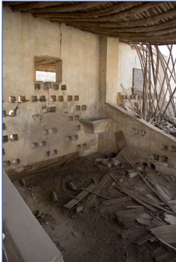
Figure 56: One of the stalls in Structure 4.
