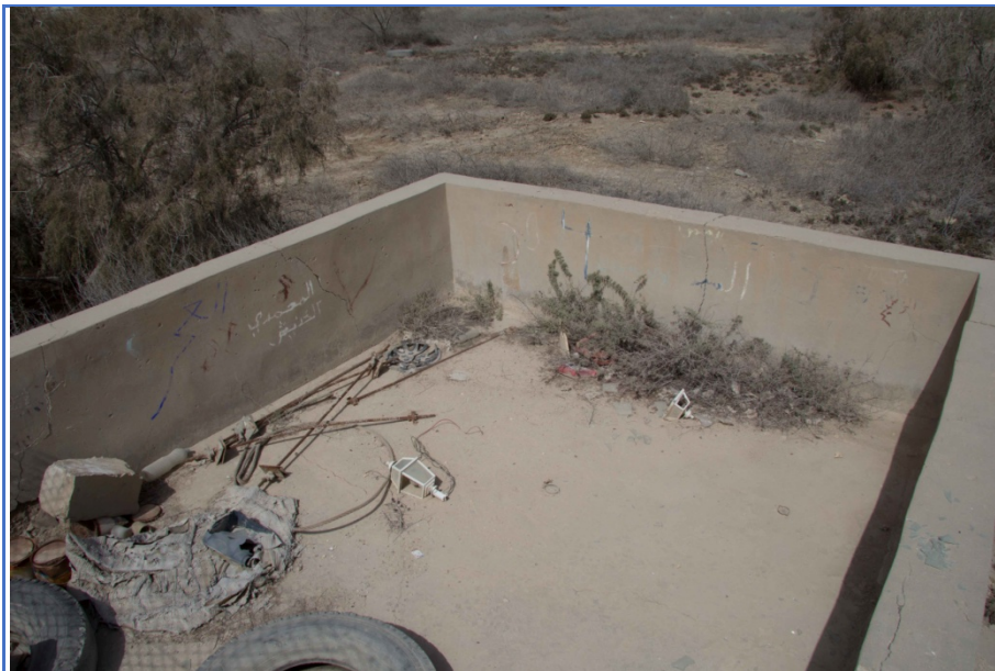
Figure 72: Raised tank located on north side of well Structure 8.
