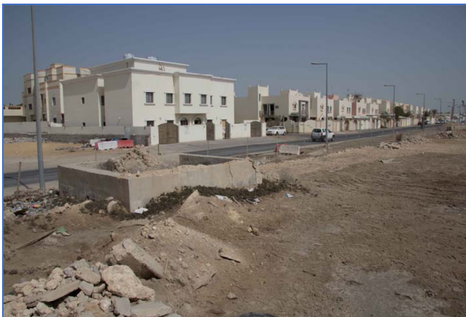
Figure 69: Concrete tank, Structure 7, looking northeast.
