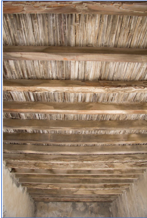
Figure 27: Square cut roof timbers in the internal space, Room 1.
