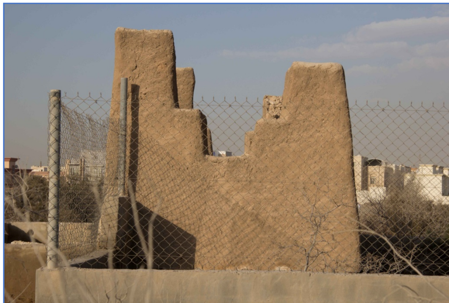
Figure 12: Photo of the east facing elevation of the well superstructure.
