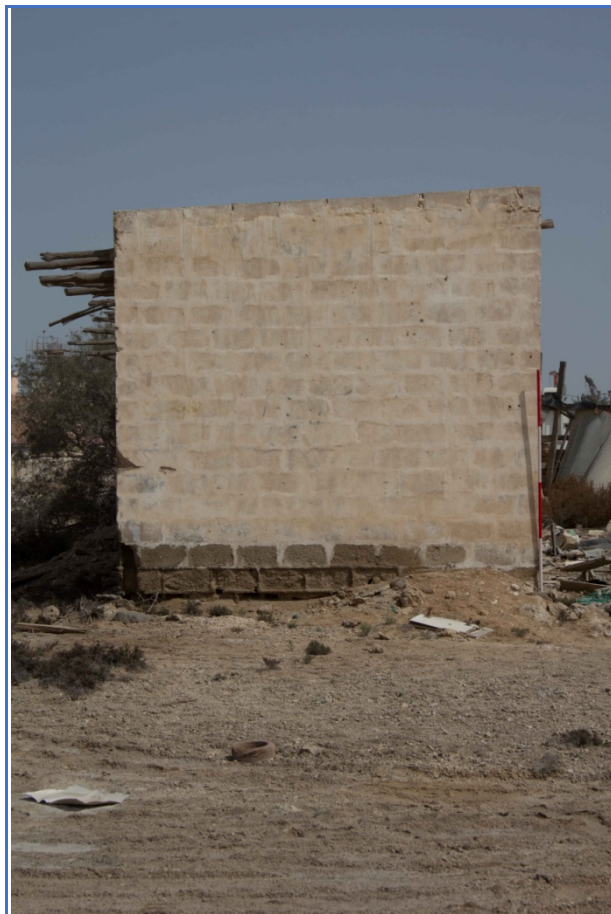
Figure 61: Photo of the west facing elevation of Structure 6.
