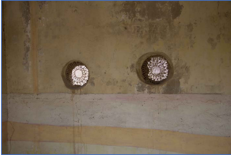
Figure 66: Ventilation holes in the kitchen, Room 4.
