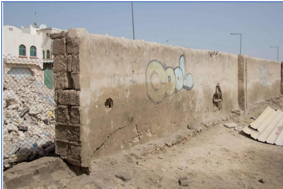
Figure 91: External wall, Structure 15.
