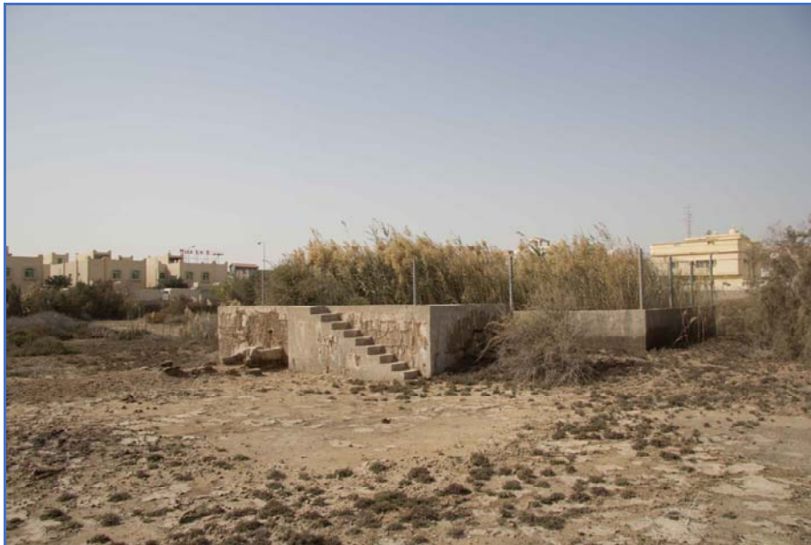
Figure 74: Steps leading up to the raised water tank with enclosed well behind, looking west.
