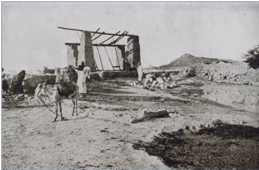
Figure 100: A traditional Zajara well in operation in Qatar, probably in the early 20th century.
