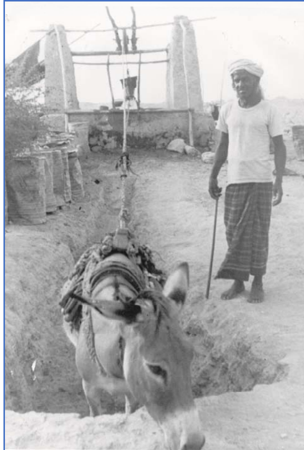
Figure 101: A traditional Zajara well in operation in Qatar, probably in the early 20th century.
