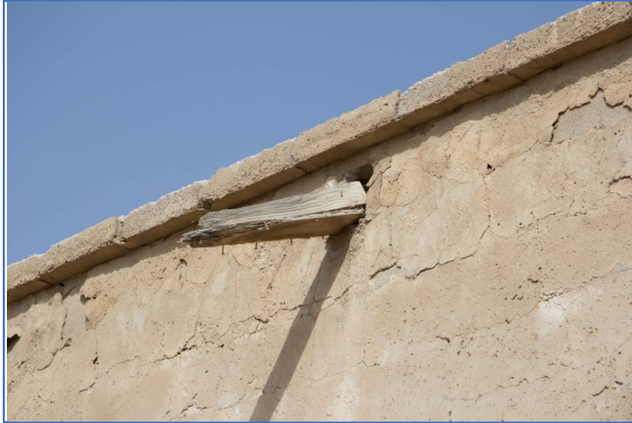
Figure 28: Water spout on the roof of the majlis.
