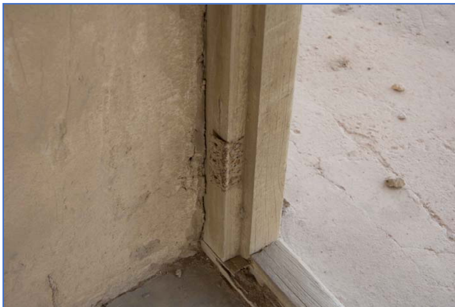
Figure 33: Detail of a surviving wooden doorframe and hinge.
