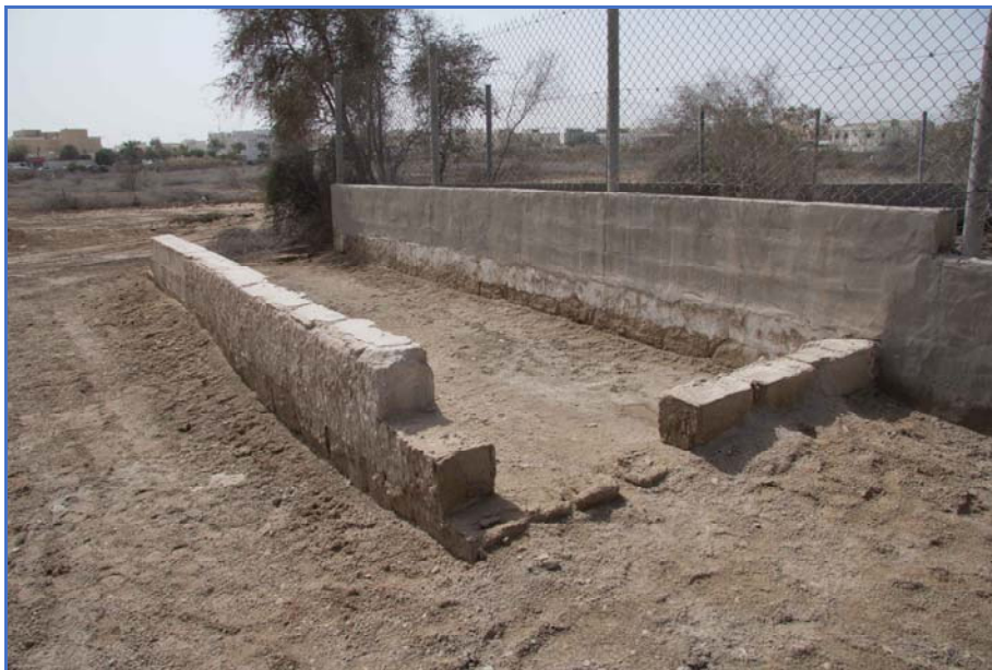
Figure 85: Water tank with enclosed well behind, Structure 12, looking southwest.
