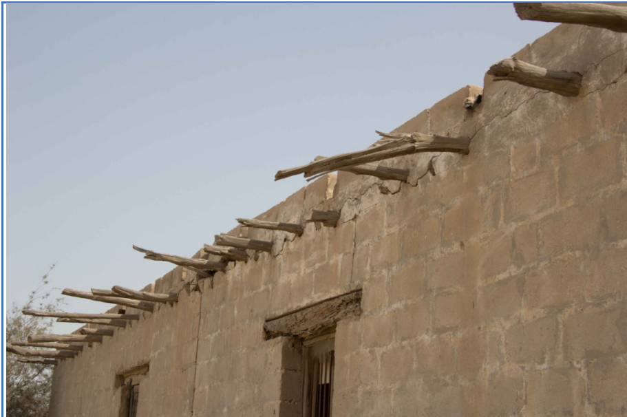
Figure 63: Danshal roof timbers extending beyond the north wall.
