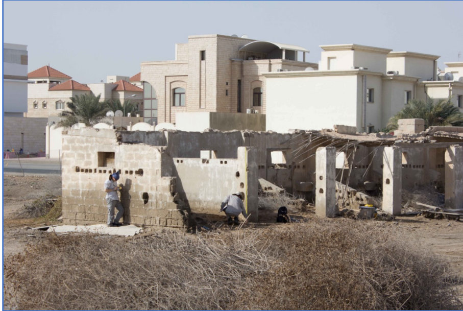
Figure 40: Ruth and Tom recording the stable block Structure 3, looking southwest.
