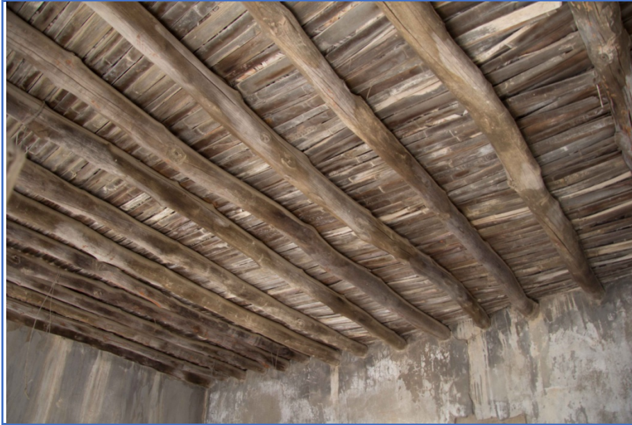
Figure 62: Ceiling and roofing timbers inside Structure 6.
