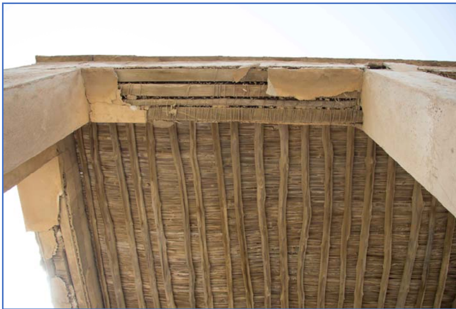
Figure 25: Detail of the construction of the colonnade.
