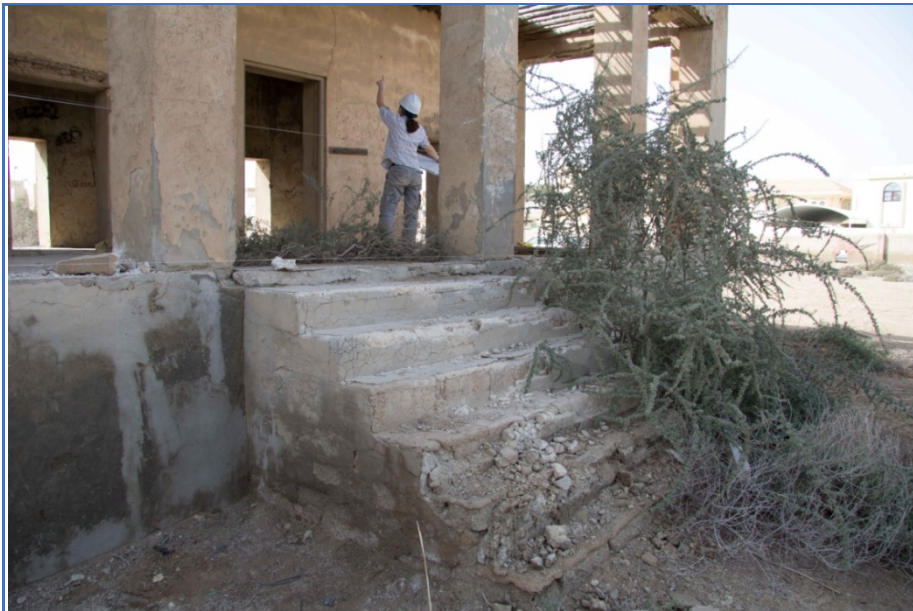
Figure 23: Stairs on the northern side of the liwan .
