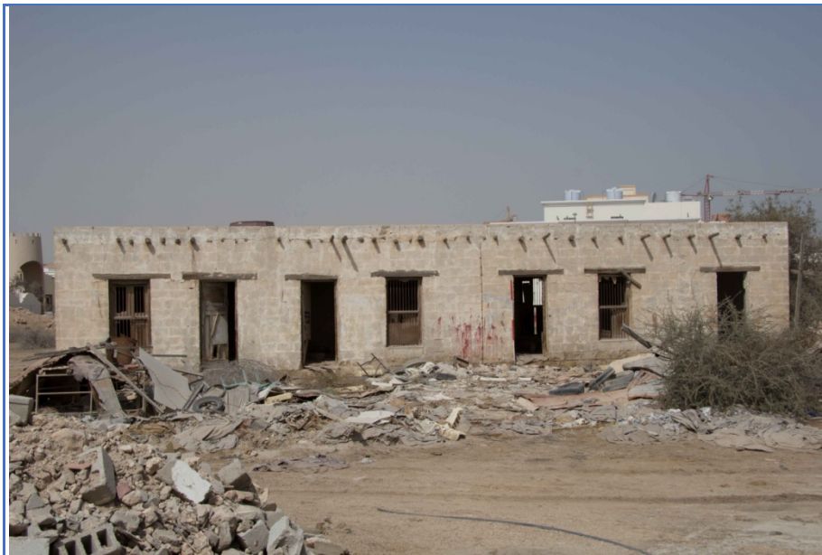
Figure 69: Photo of the south facing elevation of Structure 6.
