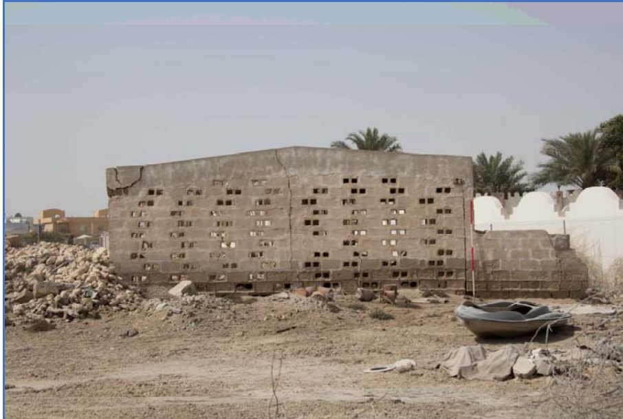
Figure 53: Photo of the west facing elevation of Structure 4.
