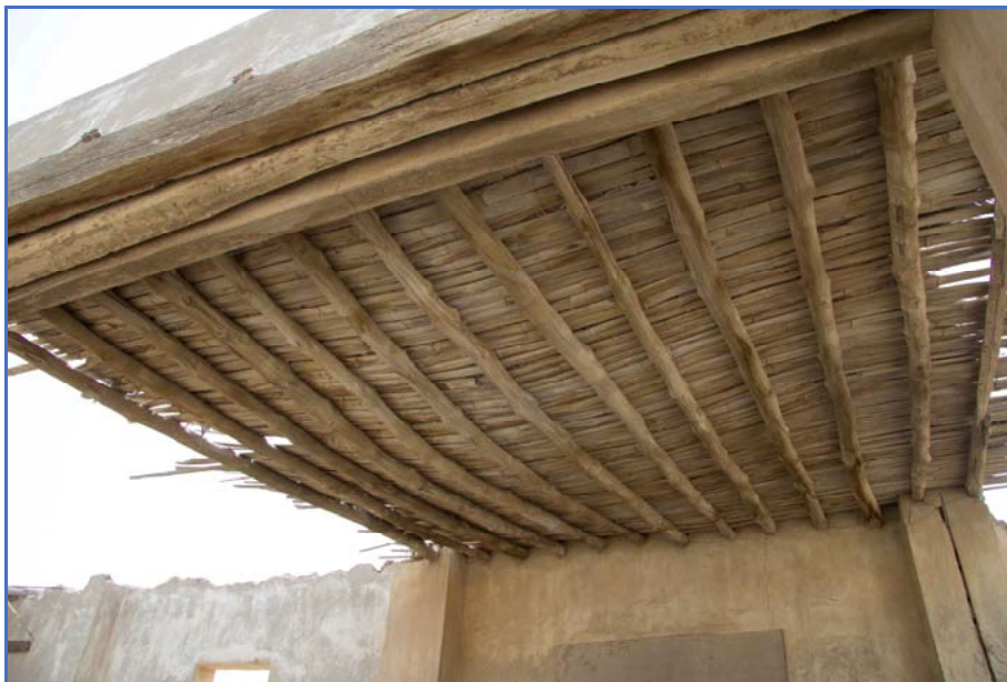
Figure 50: Traditional roofing in Structure 3.
