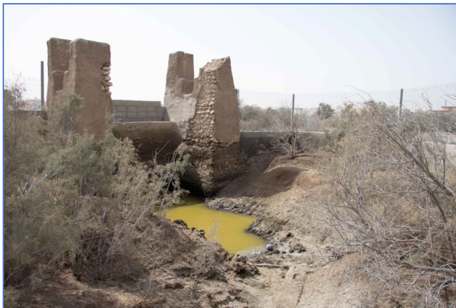
Figure 14: The well superstructure, looking northeast.
