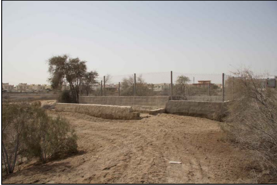
Figure 82: Water tank in foreground and enclosed well behind, Structure 12, looking southwest.
