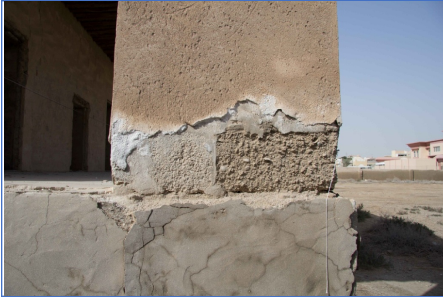
Figure 22: Shelly concrete block construction and external render
