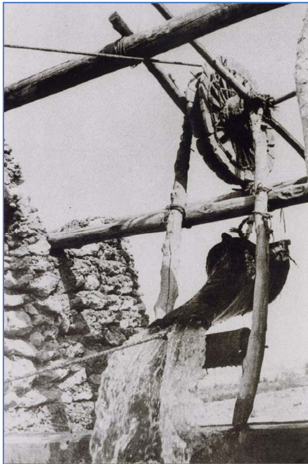
Figure 102: Detail of the leather bucket used to lift water.
